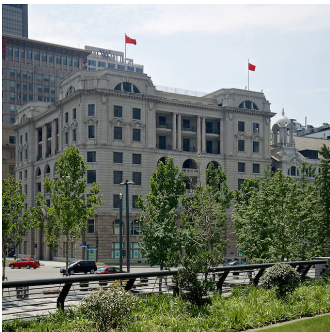
The Asiatic Petroleum Company building as it looks today
